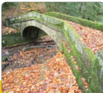
Pack Horse Bridge, Glen Howe
